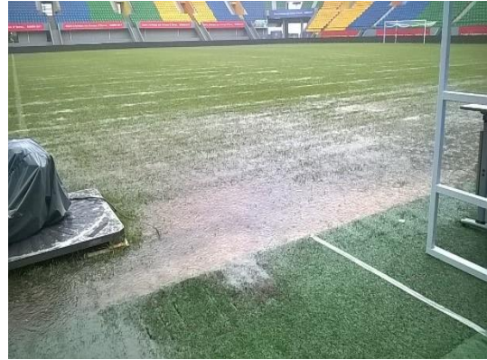
Heavy rainfall on a pitch with poor surface drainage – such conditions can lead to matches being abandoned.
