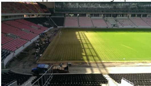
Effect of shade on turf establishment – artificial lighting rigs will be essential in winter to maintain growth.
