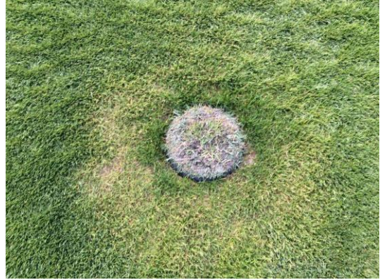
Dangerous irrigation sprinkler within the field of play.
