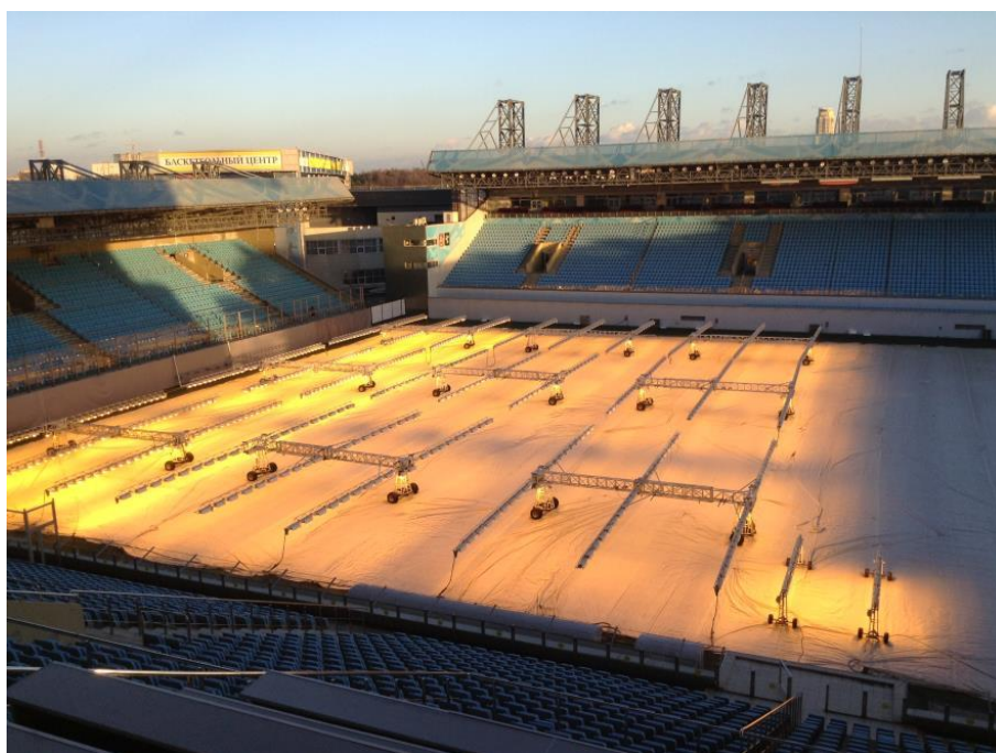
Fig. 13. Combination of lighting rigs and pitch covers.
