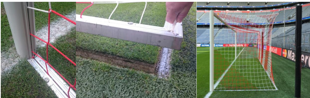
Fig. 24. Goal frames recessed into the ground.
